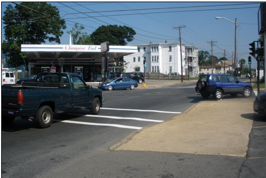
Intersection of Forest Avenue/Warren Avenue from Warren Avenue looking northbound showing pole mounted signals and multiple curb cuts
