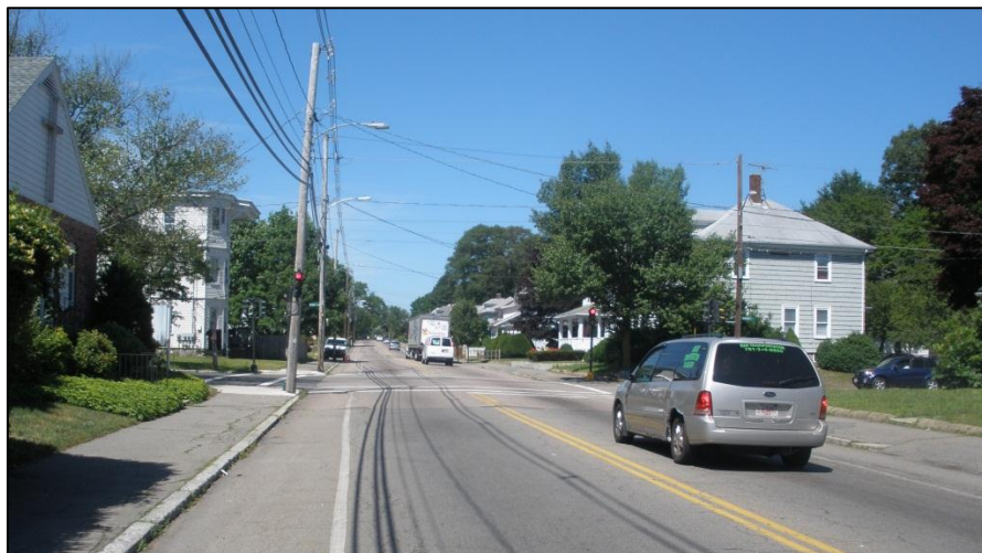
Forest Avenue looking westbound at the Bouve Avenue and Manomet Street intersection with pole mounted traffic signals set off to the side hampering visibility
