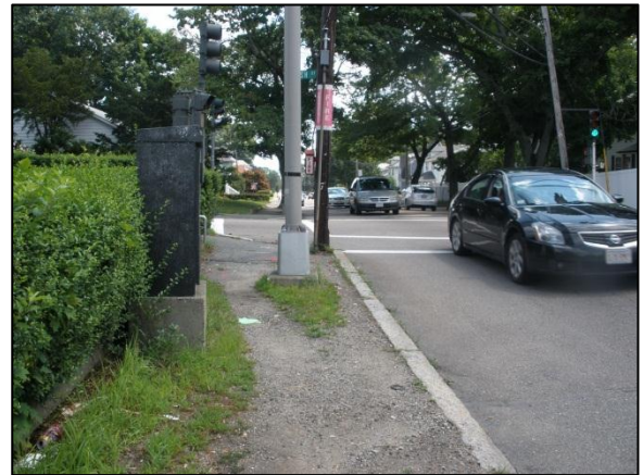
Forest Avenue at the Ash Street intersection showing overgrown vegetation impeding sidewalks, sidewalk obstacles, poor sidewalk surface conditions, and pole mounted traffic signals
