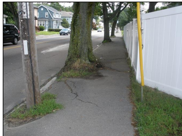
Forest Avenue in the vicinity of Ash Street with faded line denoting shoulders and poor sidewalk conditions
