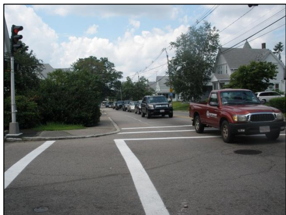
Forest Avenue at the Ash Street intersection showing overgrown vegetation impeding sidewalks, sidewalk obstacles, poor sidewalk surface conditions, and pole mounted traffic signals
