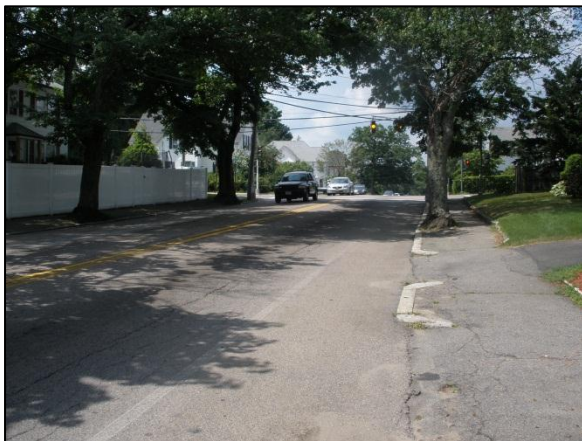
Forest Avenue in the vicinity of Ash Street with faded line denoting shoulders and poor sidewalk conditions
