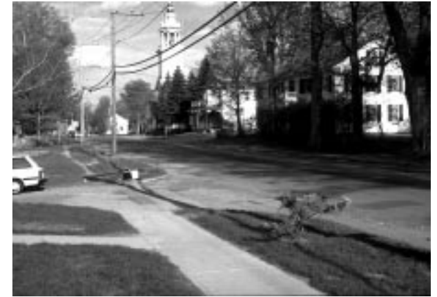
Ashfield has plans for improvements to discontinuous sidewalks along Route 116.
