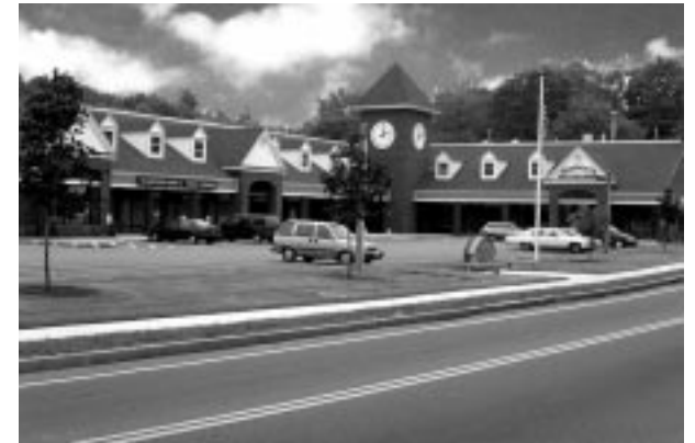
Stores can be oriented to meet the sidewalk. Walkways along storefronts connect to the sidewalk. (Littleton)
