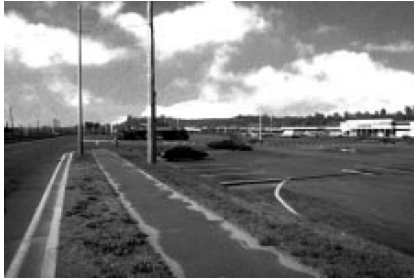
In many commercial strip developments there is no clear path between the sidewalk and stores.
