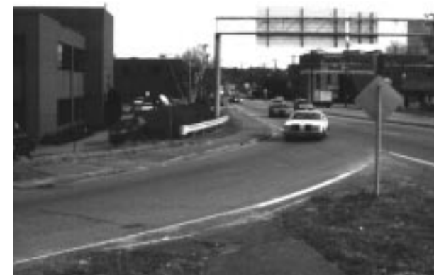
Sidewalk crossing highway ramp (Highland Ave. on-ramp to I-95 in Needham).
