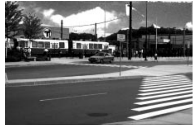
Riverside station in Newton was recently reconstructed. The new design provides clear pedestrian paths through parking areas to the platforms. At park-and-ride facilities, a balance needs to be struck between space for parked cars and walkways.
