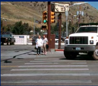
Continental Crosswalk Markings (Source: www.pedbikeimages.org )
