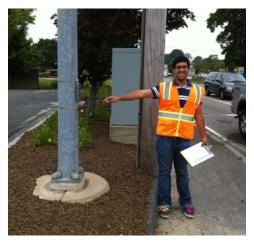
**Figure 12:** An example of an inaccessible pedestrian push button
