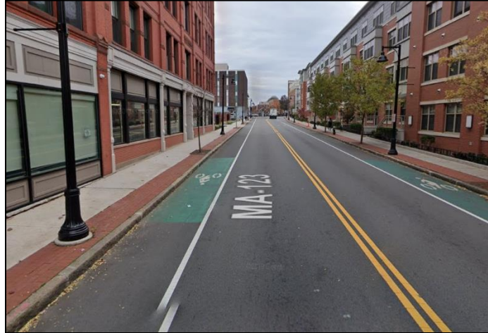
Figure 28 Bicycle lanes on Centre Street in Downtown Brockton.
