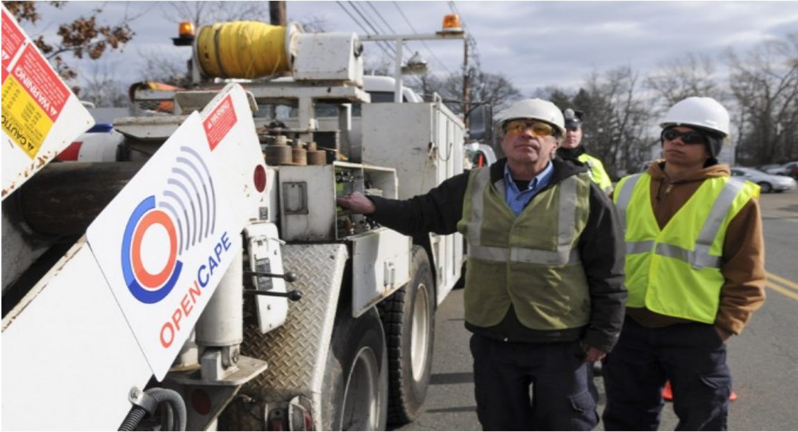
OpenCape cable laying machine
