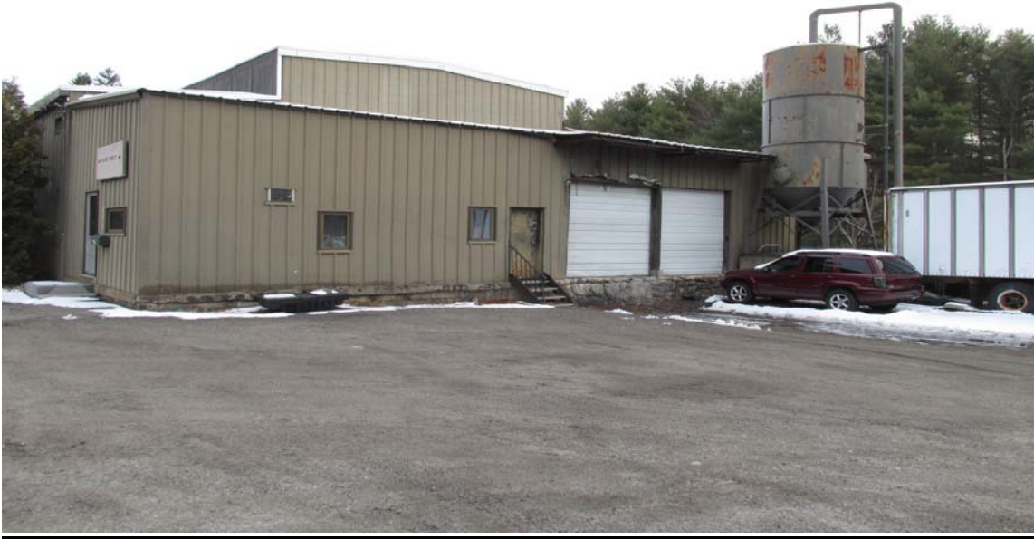
KolTar Abington plant
