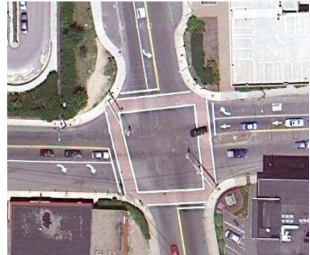
Commercial and Centre Streets Brockton, MA
