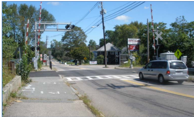
Plymouth Street with crosswalk and stop line to the west of the railroad grade crossing and stop line on the east side of the railroad tracks
