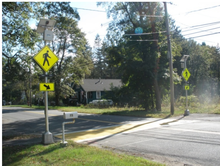
Rapid Rectangular Flashing Pedestrian Warning Signs
