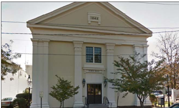
Bridgewater Town Hall in Central Square
