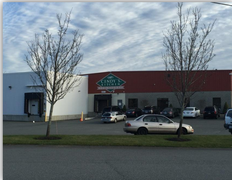
Figure 3-2: Cindy's Kitchen Manufacturing Facility
