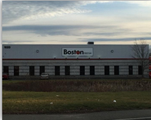
Figure 2-2: Boston Fresh Distribution Facility
