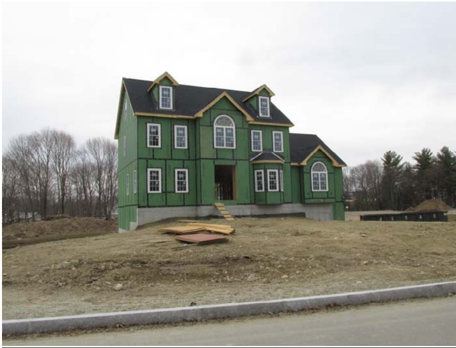
Single family home under construction in Abington, April 2018
