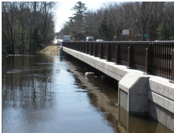
Figure 3.24: Route 18 spanning the Taunton River in Bridgewater, March 2010
