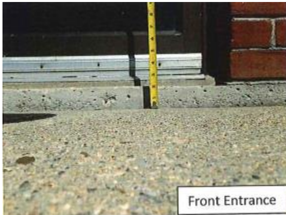
Figure 63: Pembroke Fire Station Main (front) Entrance
