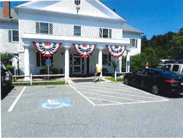
Figure 36: Pembroke Town Hall
