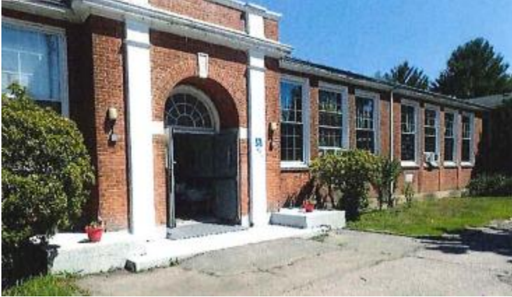
Figure 44: Pembroke Recreation Center
