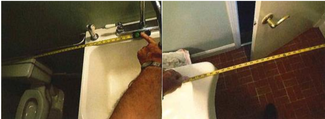
Figure 57: The COA public unisex toilet room.
