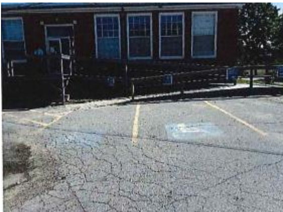
Figure 46: Switchback wood access ramp
