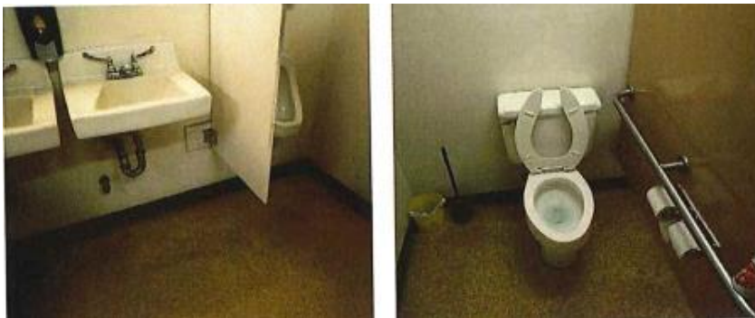
Figure 64: Fire Station Men’s Restroom
