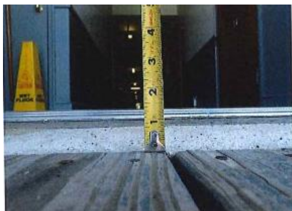
Figure 47: Gaps between planks and deteriorated, irregular concrete
