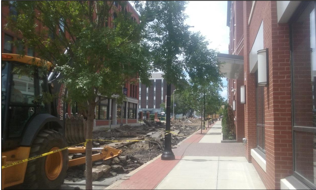
Figure 10 Centre Street Reconstruction in Brockton
