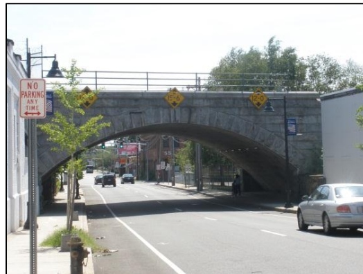
Crescent Avenue (Route 123) looking eastbound toward the Historic Stone Arch Bridge
