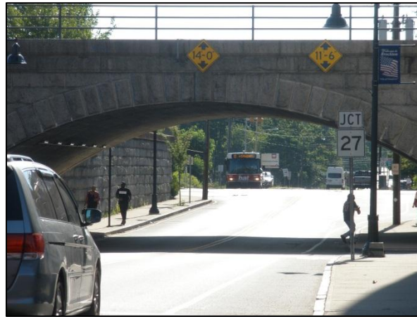
Centre Avenue (Route 123) looking eastbound toward the Historic Stone Arch Bridge
