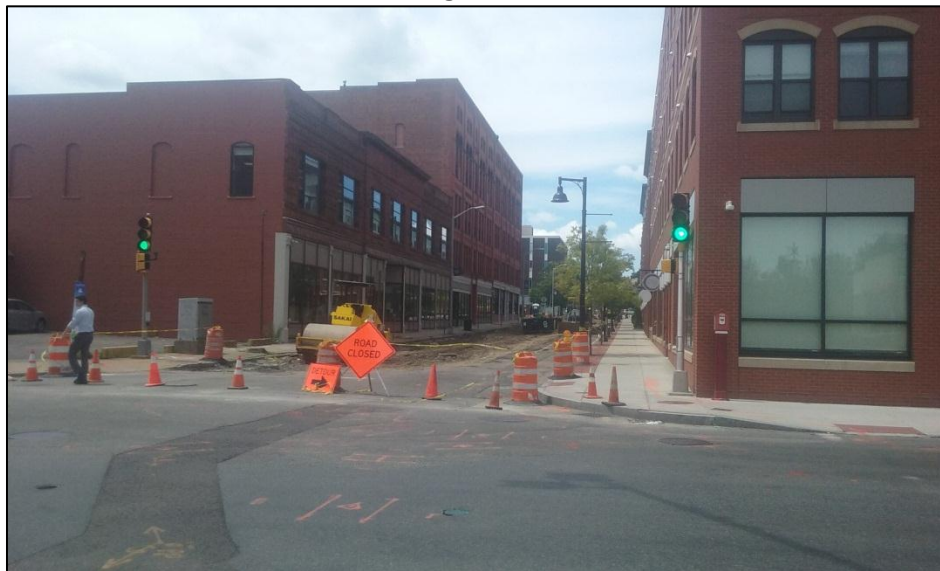
The Reconstruction of the Centre Street (Route 123)/Montello Street (Route 28) intersection
