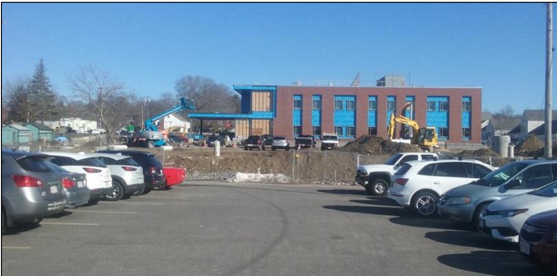
Signature Health Care (Brockton Hospital) New Cancer Center under construction
