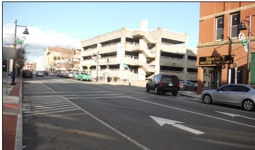
The Main Street/Crescent Street (Route 123) intersection showing two through lanes, exclusive northbound right turn (green arrow), and lack of overhead signal heads
