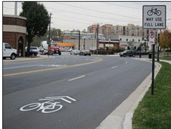
Sharrows for Bicycle Accommodation
