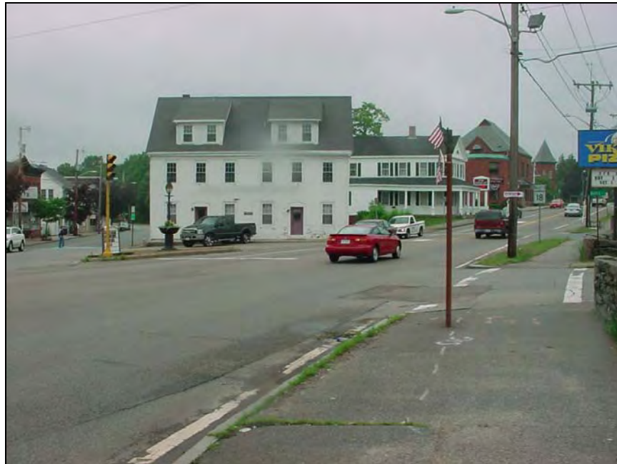
East Bridgewater Center looking north toward mid-block crossing on Route 18
