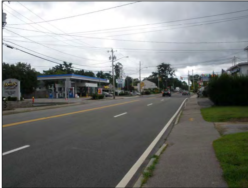
Resurfacing Route 18 in Whitman at the Route 27 intersection
