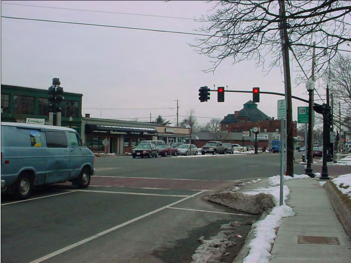
Stoughton Square looking northbound showing pedestrian bump-outs, crosswalks, and upgraded traffic signals.
