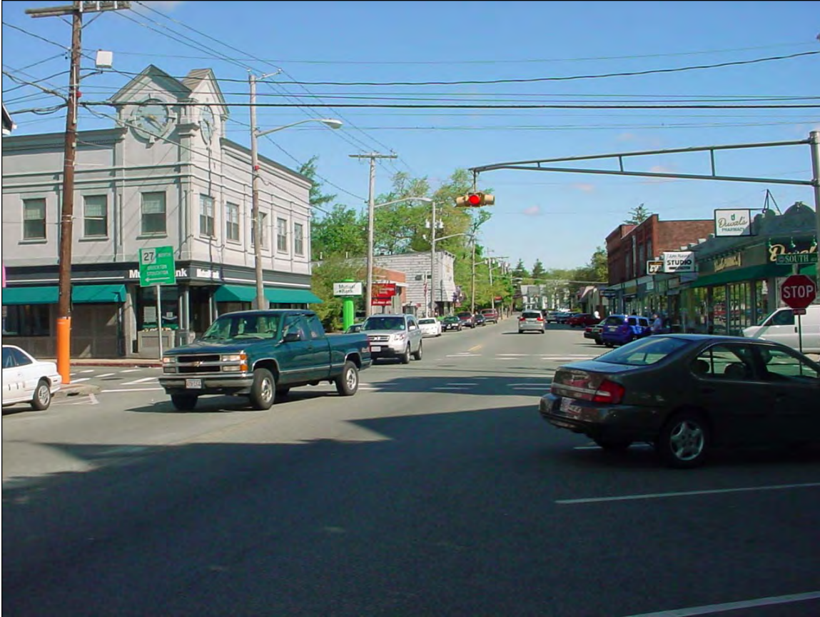
Route 27 (Temple Street)/South Avenue/Washington Street intersection at Whitman Center looking north from the Washington Street approach.
