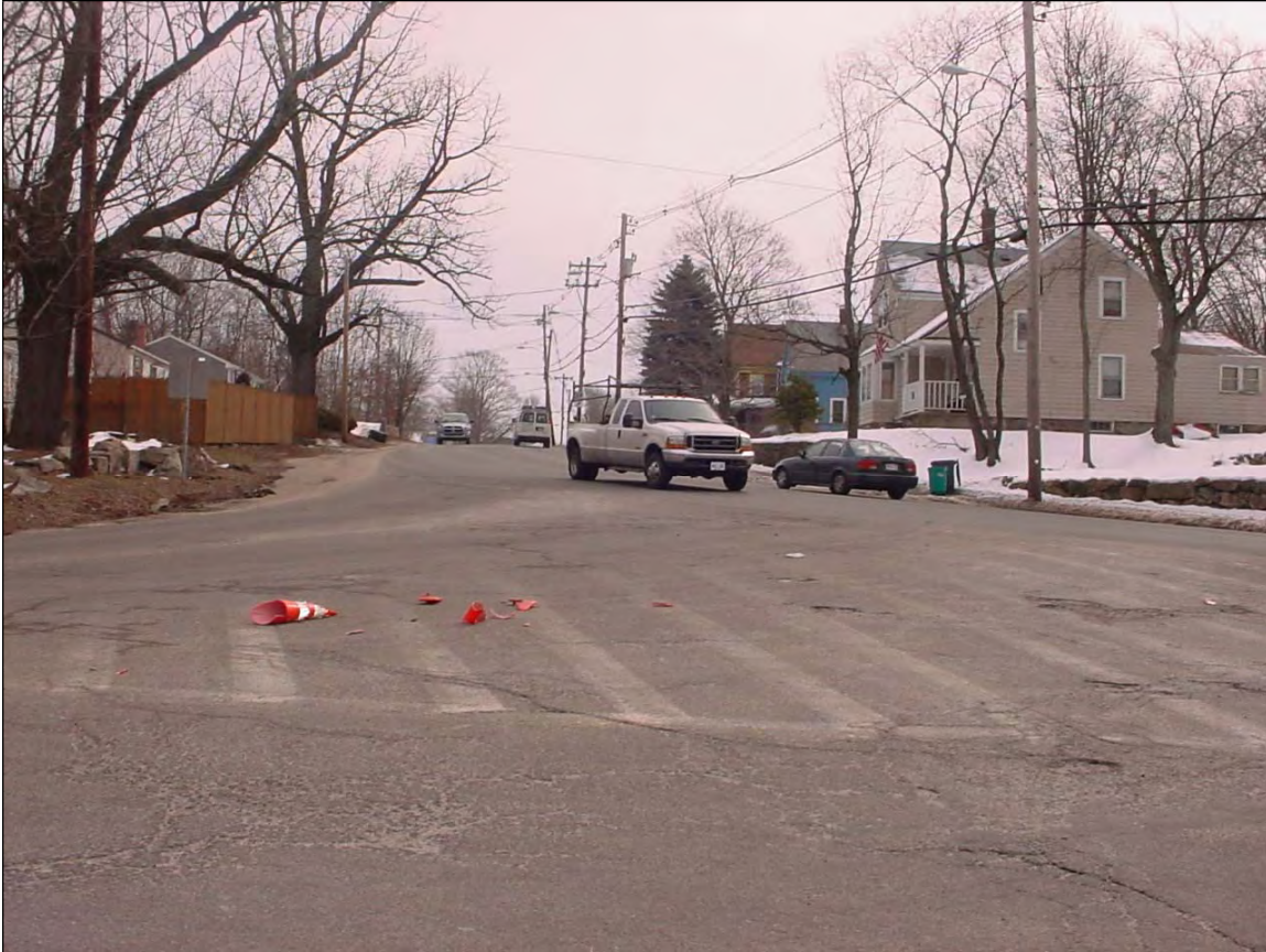
The Route 27 (Central Street)/Island Street intersection looking east, showing the faded pavement island on the Island Street approach.
