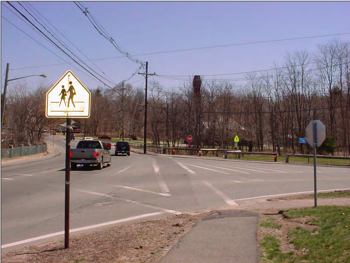
The Route 27 (Central Street)/West Street intersection looking east showing the approximately 110 foot long crosswalk and faded pavement island on the West Street approach.
