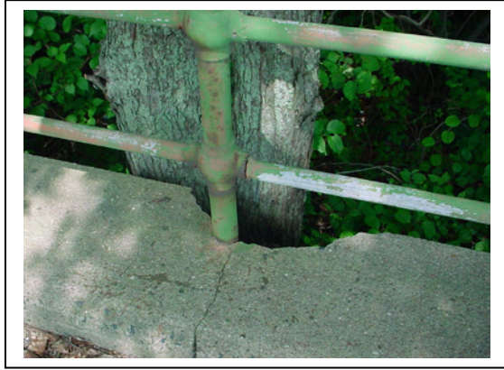
Figures 3, 4, and 5: Images show railing systems in disrepair and structural cracking and crumbling on bridges over the Jones River and water-flow between Jones River and Foundry Pond.
