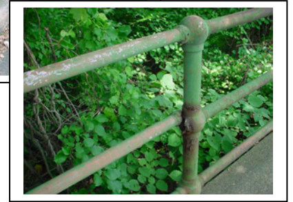
Figures 3, 4, and 5: Images show railing systems in disrepair and structural cracking and crumbling on bridges over the Jones River and water-flow between Jones River and Foundry Pond.
