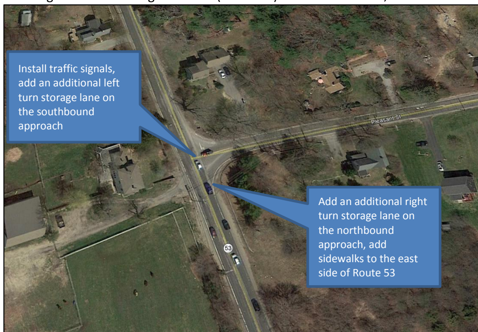
Figure 15 – Washington Street (Route 53) at Pleasant Street, Pembroke
