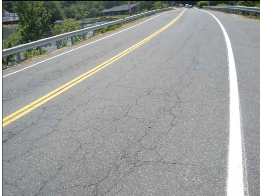
Route 58 pavement conditions in Halifax at West Monponsett Pond and East Monponsett Pond looking north (Poor conditions).
