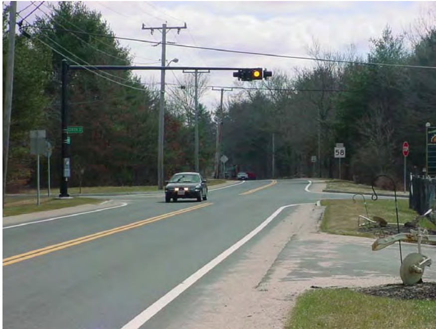
Route 58, Plympton at Center Street showing completed improvements that include re-stripping, pavement resurfacing, and installation of a flashing beacon.
