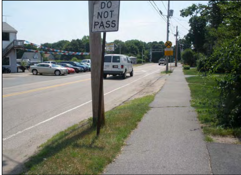
Route 58 in Abington looking south toward the Railroad tracks showing typical sidewalk on the southbound side with a grass buffer but no raised curbs.
