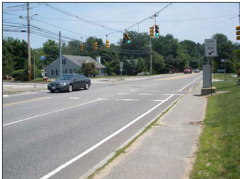
Sidewalks at the Route 58/Winter Street intersection in Hanson looking south.
