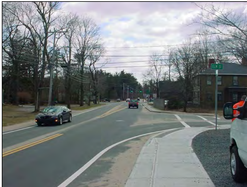
Route 58 sidewalks in Plympton near Elm Street and Parsonage/Mayflower Road
