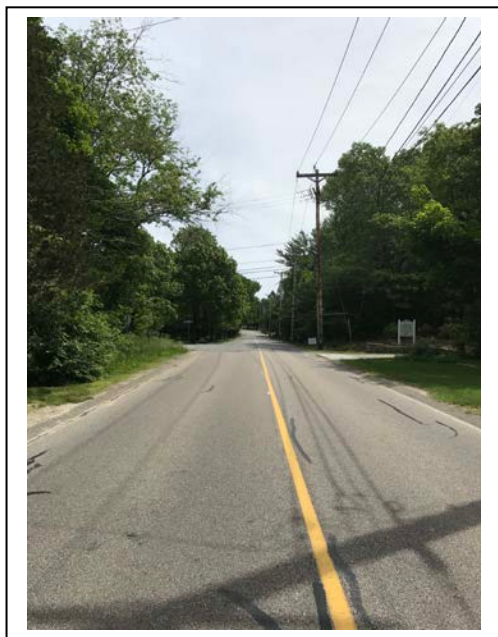
Figure 3: Alden Street at Railroad Avenue
