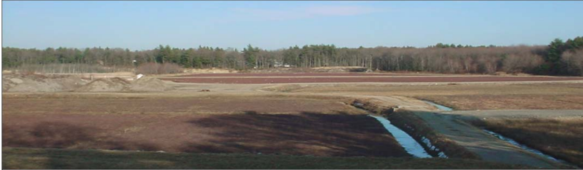
Figure 3-19: The Wampatuck Bogs viewed from Robinson Street - formerly abandoned and now being restored in Hanson
