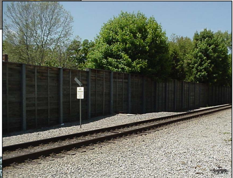
Figure 6-11: Commuter Rail Sound Proofing
