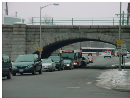
Figure 3-15: Rail Bridge over Route 27 in downtown Brockton
