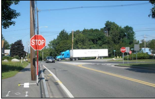
Figure 5-5: A tractor-trailer truck exiting Tosca Drive encroaches on the Central Street (Route 27) eastbound travel lane
