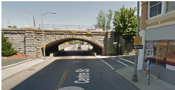
Height limitations on Centre Street (Route 27) Brockton – 14.0 feet at the center, 11 feet 6 inches at the edge of the road
