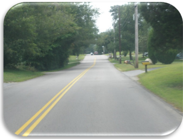
Figure 3: East Street, Bridgewater, MA
