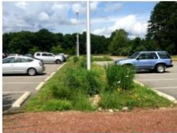
Bioretention strips filter parking lot runoff
