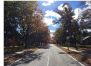
This narrow road in Devens, MA easily fits two lanes of traffic and offers room for a vegetated buffer, sidewalk, and street trees.
