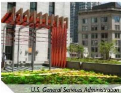
U.S. General Services Administration Boston, MA: John W. McCormack US Post Office and Courthouse. This 9,654 ft 2 green roof sits atop the EPA Region 1 Headquarters on a historic 1933 building.
