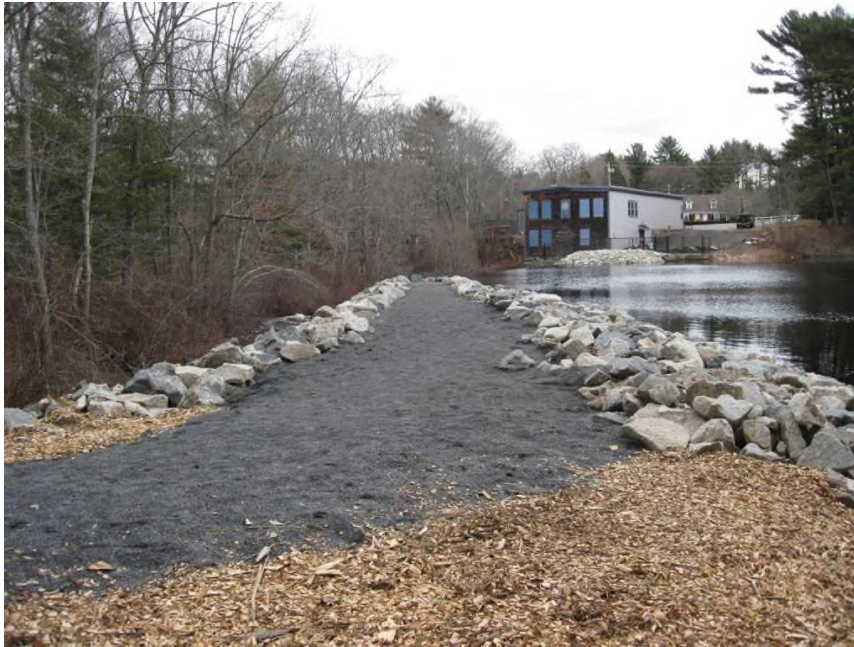
Dam Crest from left abutment Construction Completed 2015
