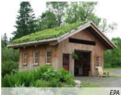
EPA A small, slanted green roof in Craftsbury, VT.
