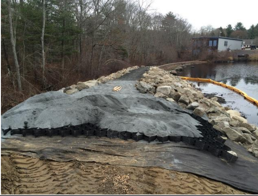
Figure 43: Factory Pond Dam, during repair work
