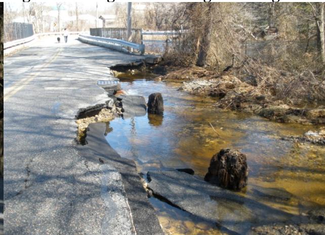
Figure 7: Bridge Street Bridge in Bridgewater
