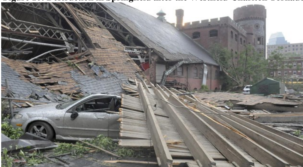
Figure 10: Destruction in Springfield after the Westfield-Charlton Tornado
