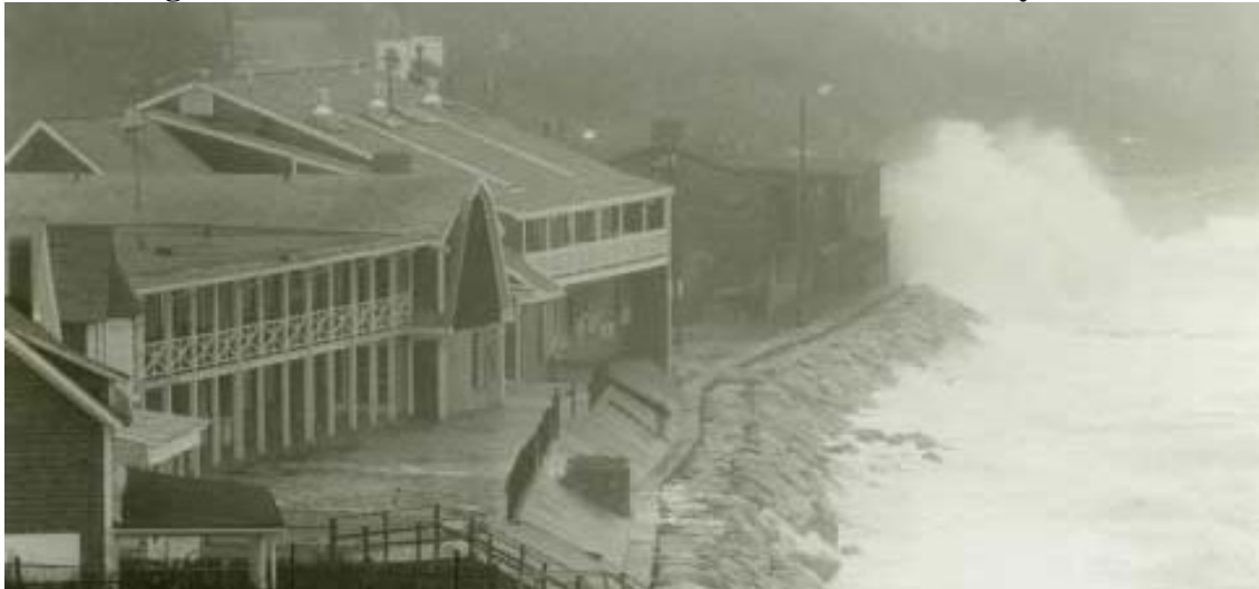
Figure 14: Coastal Erosion from the “Perfect Storm” in Plymouth
