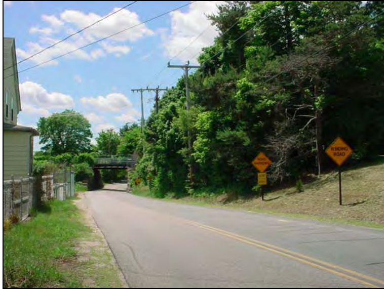
Landing Road looking southbound toward the MBTA Bridge
