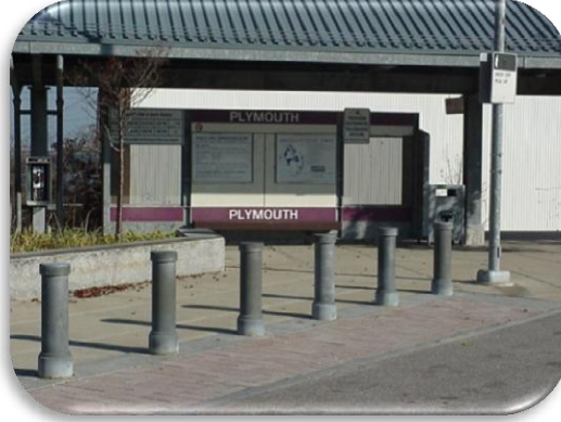
Figure 2.15: MBTA Commuter Rail Station, Plymouth
