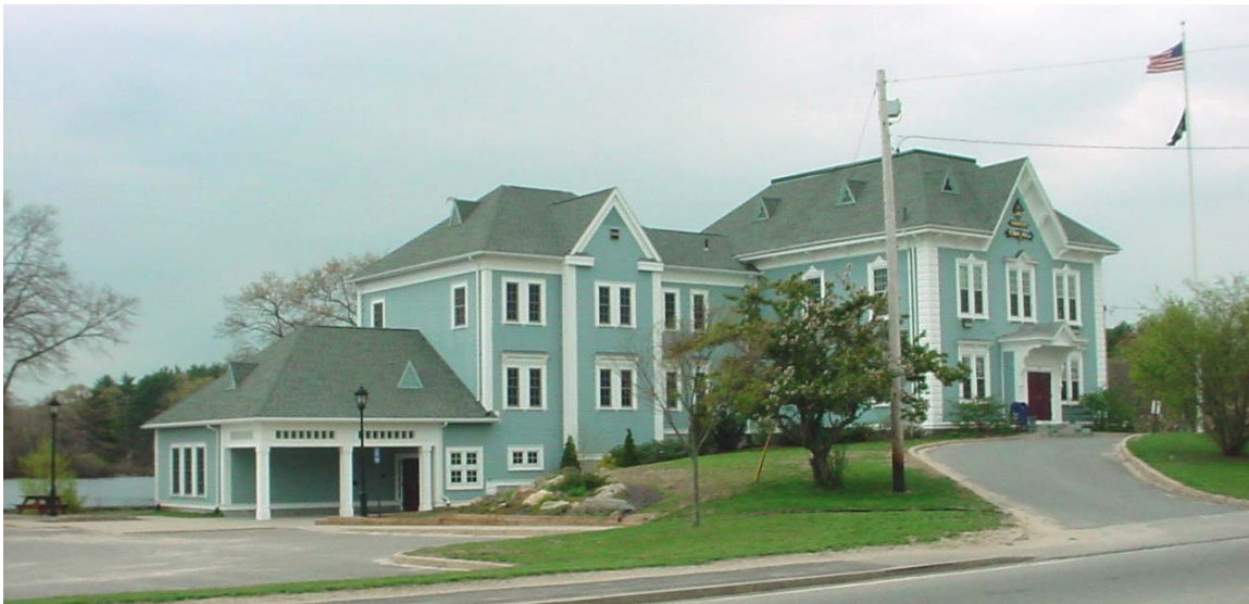
The recently enlarged Town Hall - minus its prior black iron roof ornamentation
