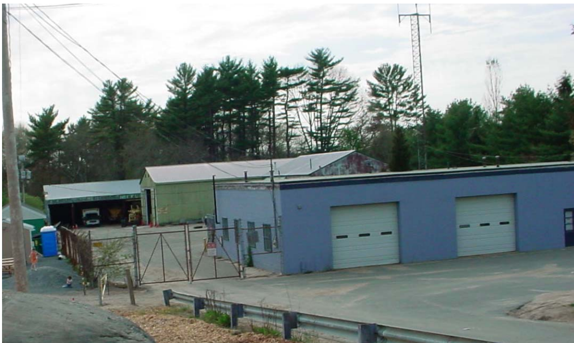
The Highway Department's Town Barn Complex behind the Police Station
