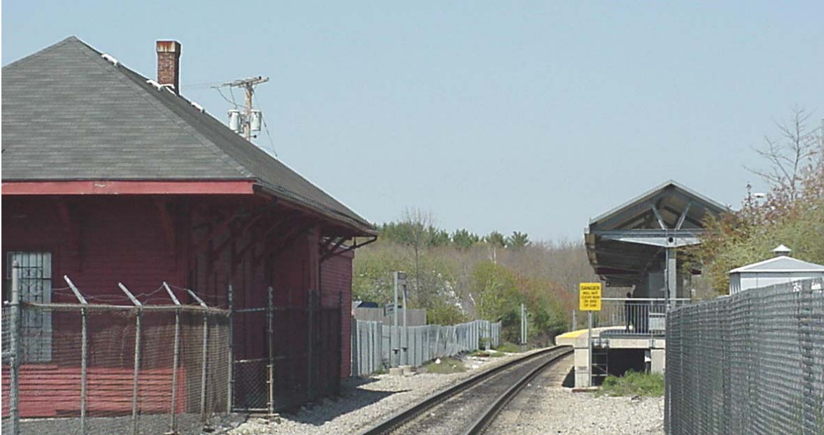
Intact, but unused old South Hanson Station (left) across from new station's minimal shelter
