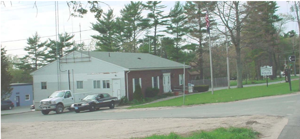
Present Police Station - soon to be replaced by a bigger station on Route 27.
