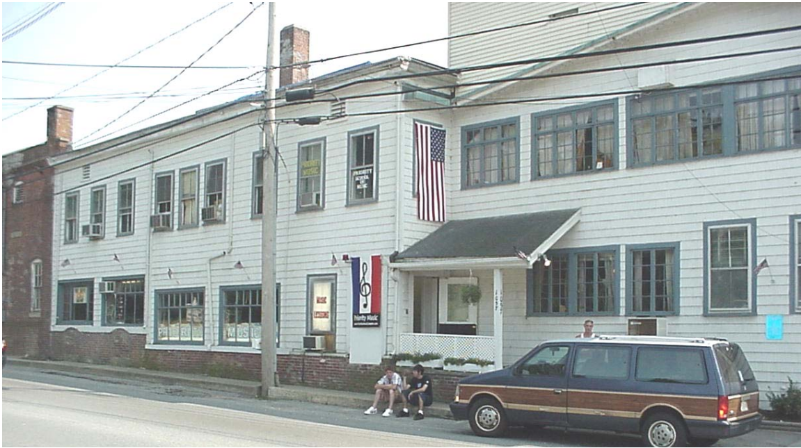
South Hanson - Older buildings in Current Use - fully occupied by music businesses and studios.
