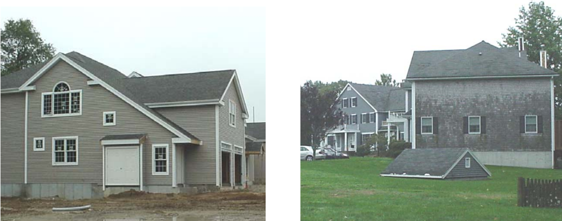
Dunham Farms under construction (left) and abutting market rate multi-unit housing (right) at corner of Main and High Streets at the edge of the proposed TOD-I District
