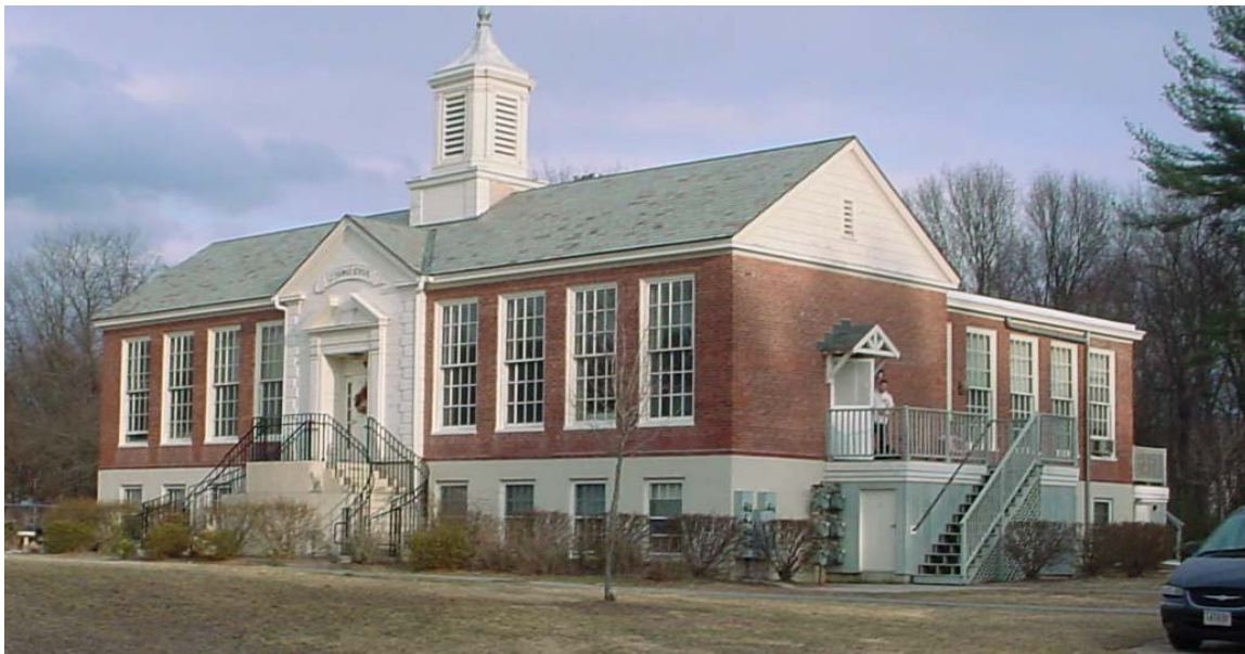
1929 L. Z. Thomas School, converted to family housing by the Hanson Housing Authority. Note resident on typical second floor deck.
