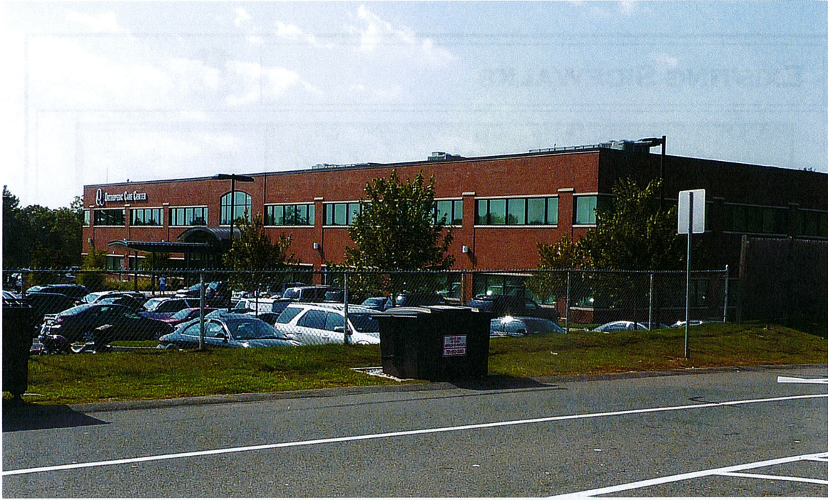
Fence along driveway behind retail building precluding a direct walk to the medical office building
