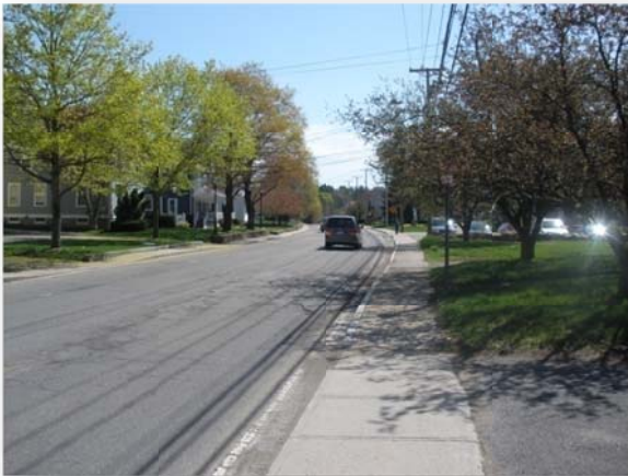
Main Street looking eastbound
