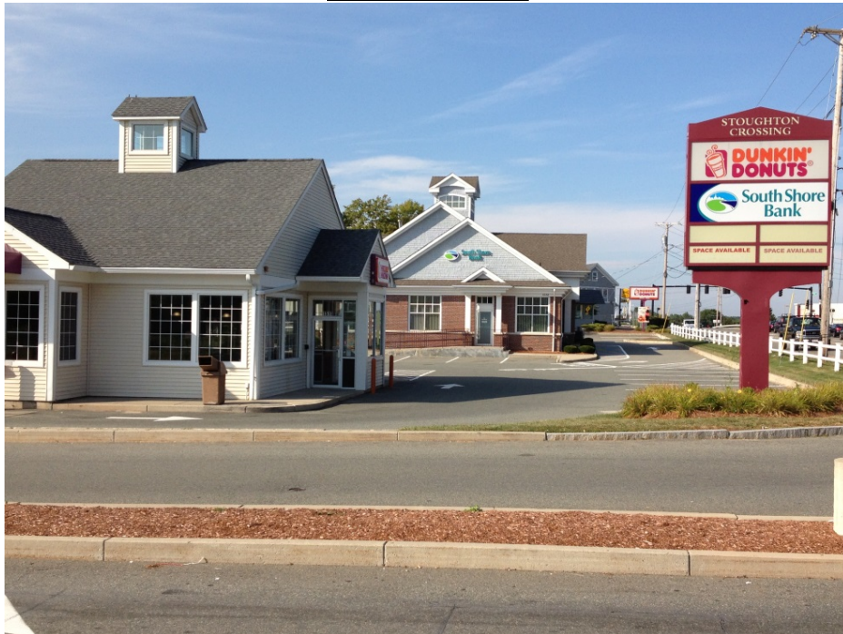
Dunkin Donuts and South Shore Bank, 1516-1538 Turnpike Street
