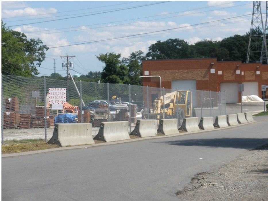
Page Building Construction & Canton Masonry, 135 Old Page Street
