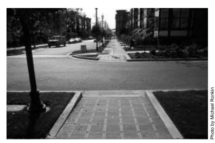
A curb ramp should be designed to provide direct access and should have the proper width and slope.
