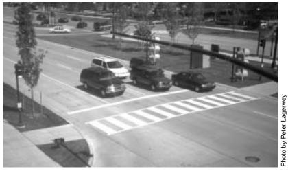
The "ladder" pattern shown above is more visible to motorists than parallel lines and requires less maintenance if painted to allow the tires of motor vehicles to track between the painted lines.
