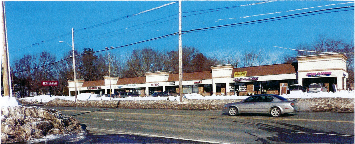
D'Angelos Strip Mall east side of the southern end of Route 138 with two curb cuts for many businesses
