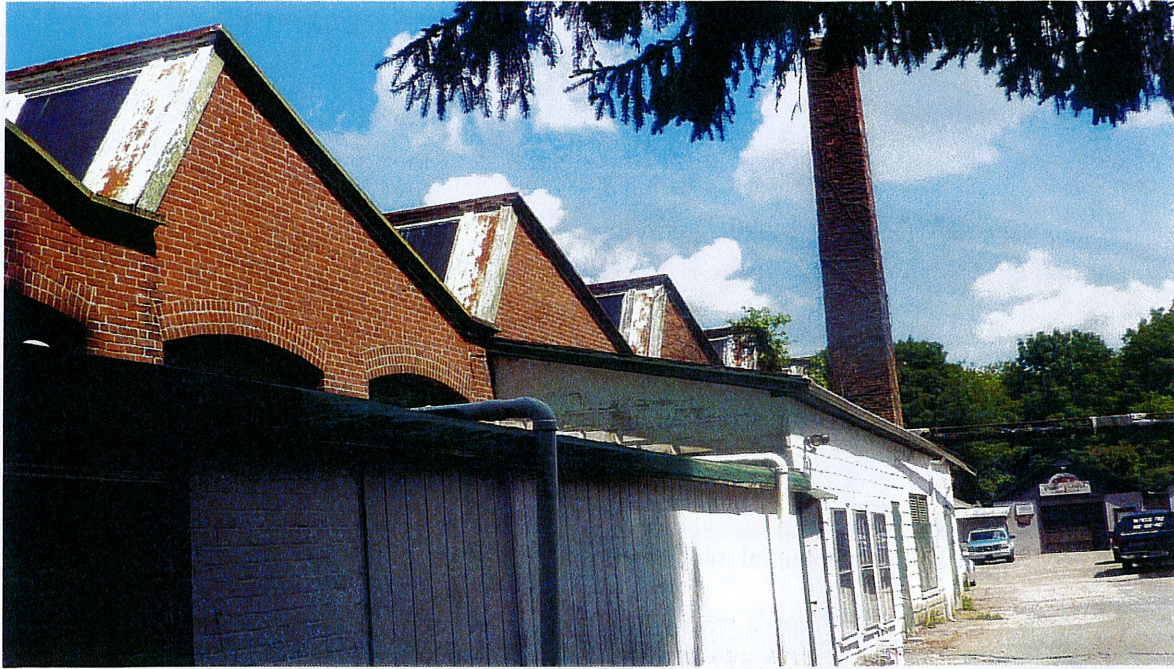
Traditional north facing skylights in Crowfoot Gear Works building-suggesting re-use for studios?
