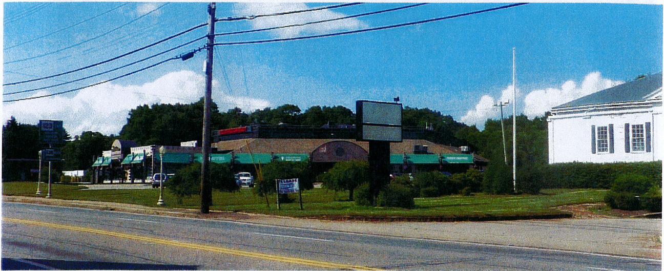
Little used land between buildings; a potential in-fill site?
