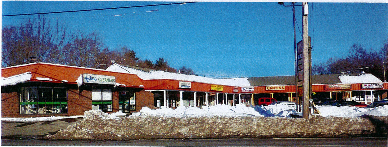
Multi-tenant Easton Plaza on Route 138; fewer curb cuts and some presence on the street frontage
