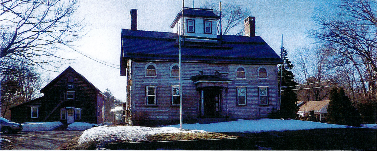
Landmark House at northwest corner of study area- a potential office conversion?
