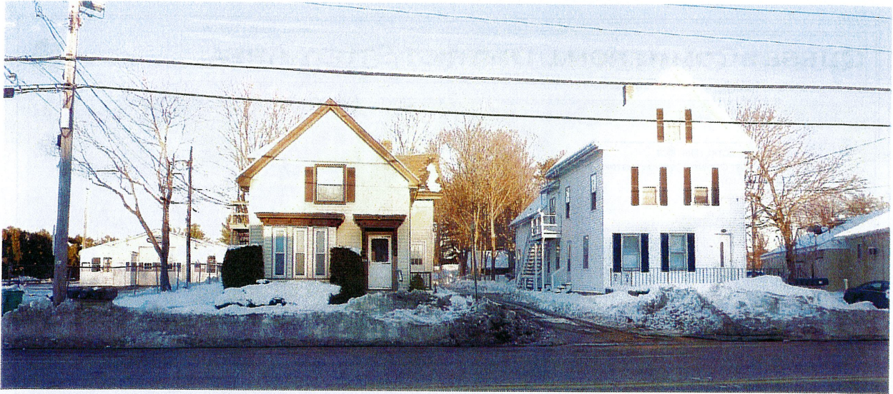
Remaining houses on Washington Street with a repair garage to the rear.
