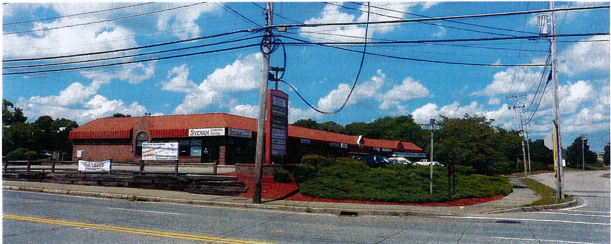
Multi-tenant building at corner of Plymouth Drive; just two curb cuts for nine businesses
