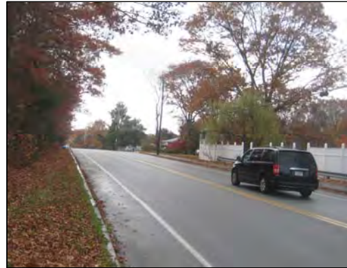
Sight distance to the south of Chestnut Street is obscured by a vertical curve on North Quincy Street.
