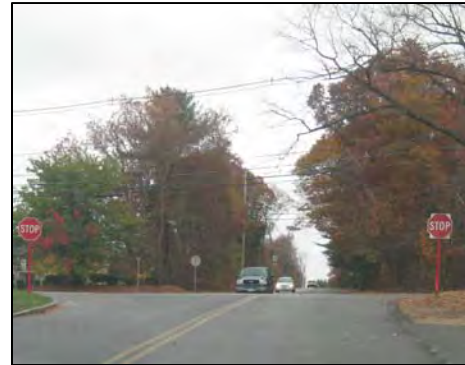
A square sign on the back of one of the two Boundary Avenue eastbound stop signs obscures the stop sign's octagonal shape.
