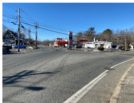
Image 1: Image shows Rockland Street Stop Line set far back from travel lane of Brockton Avenue, and proximity of gas station curb cuts to intersection.
