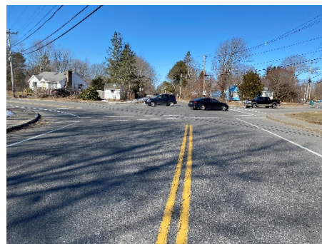
Image 2: Crosswalks do not have accessible ramps. Crosswalk across Route 139 is long, leaving pedestrians exposed.
