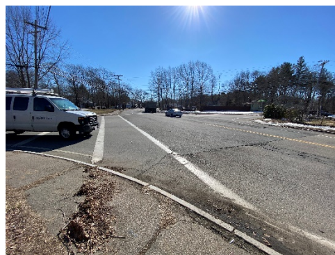
Image 1: Intersection has skewed geometry, with Old Randolph Street coming into intersection north of Chestnut Street.
