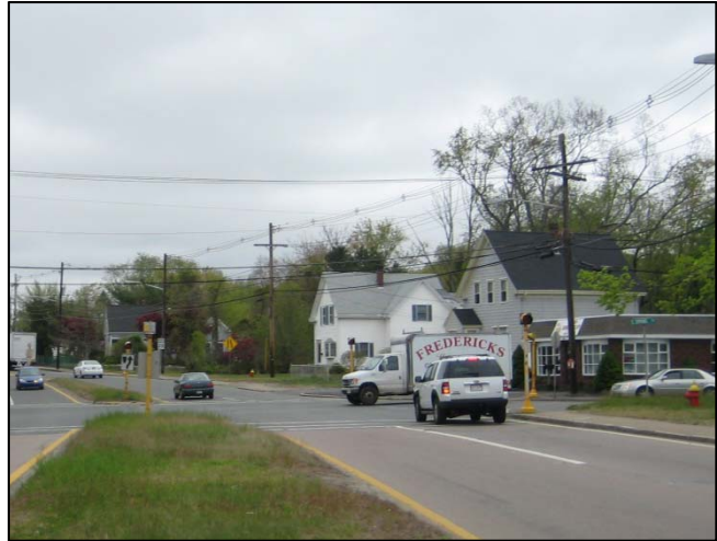
“De facto” right-turn lane along Route 28 northbound adds to driver confusion.
