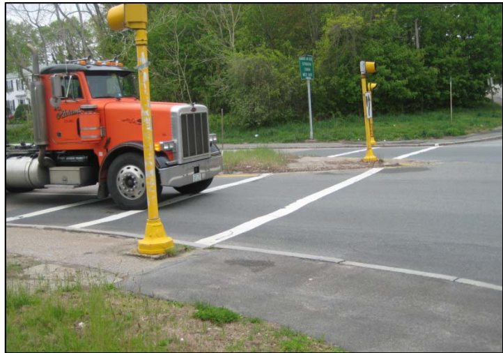
Accessible curb ramps are not provided across Route 28.
