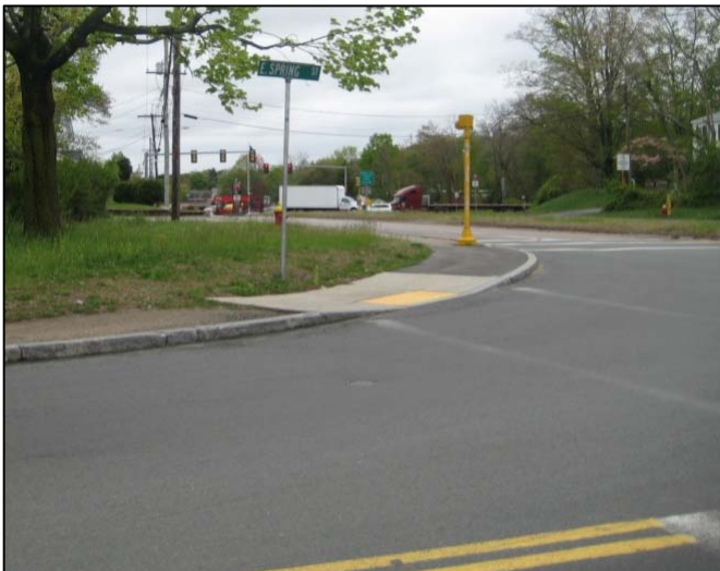
Limited sight lines south of intersection due to crest vertical curve in Route 28.
