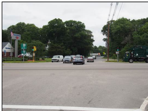
Figure 14 - Pond Street eastbound approach with pedestal mounted signals
