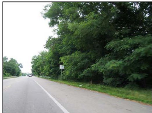
Figure 7 - Vegetation along the north side of Harrison Boulevard partially obstructing sign visibility
