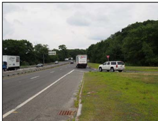
Figure 9 - Route 24 northbound exit ramp terminus at Harrison Boulevard
