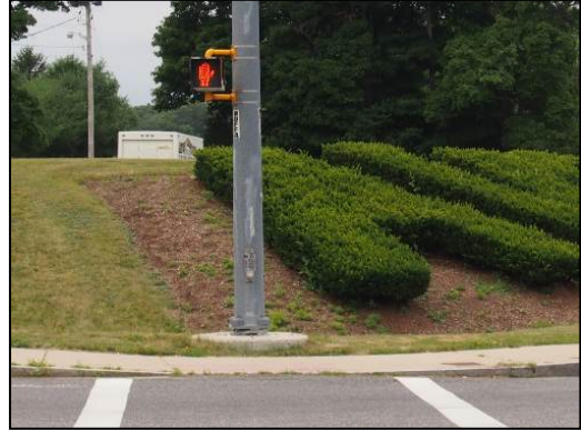
Figure 16 - Pedestrian signal indication and crosswalk
