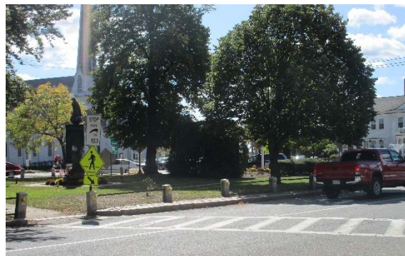
Image 4: Central Square Pedestrian Crossing Providing Non-Compliant Signage
