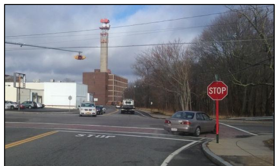
Vegetation to the right of the photo (northeast corner) obscures sight distances for vehicles waiting at stop line on the southbound approach
