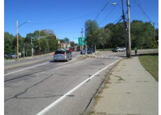
Figure 13: Looking East on Crescent Street Right Turn Lane
