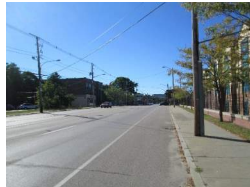
Figure 16: Looking West on Crescent Street (Plouffe School)
