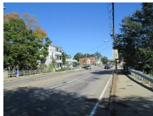
Figure 10: Vegetation to the East inhibiting Fire station egress sight distance
