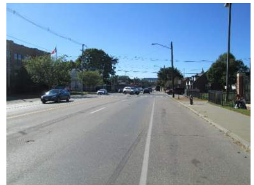
Figure 17: Looking West on Crescent Street
