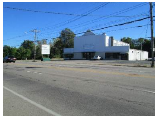
Figure 9: Looking South at the Church
