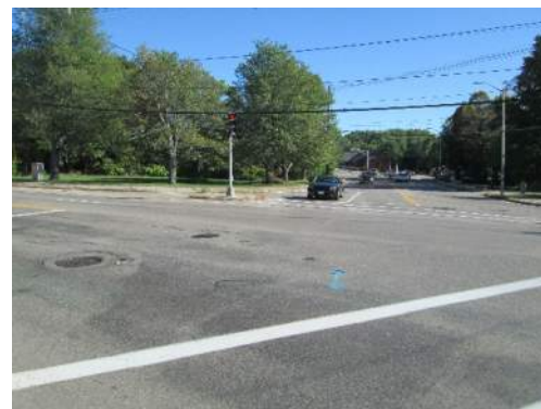
Figure 12: Looking South down Summer Street
