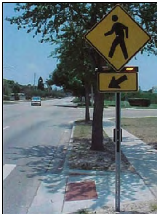
Flashing lights on the W-11 sign (Rectangular Rapid Flashing Beacons - RRFB), used in conjunction with a crosswalk. These lights are pedestrian push-button actuated.
