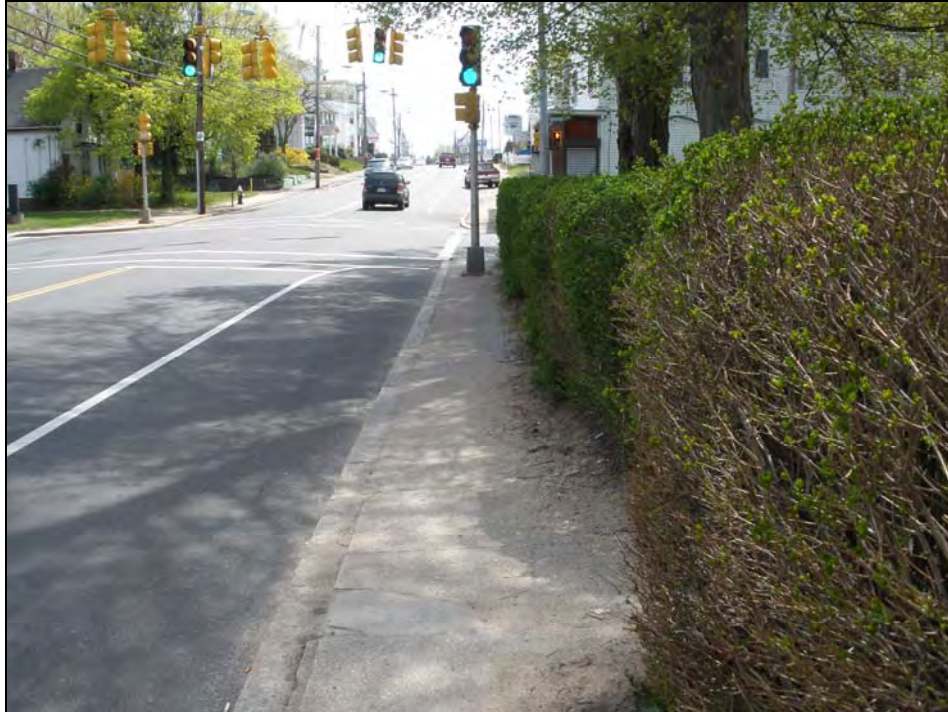
Main Street looking south at Brookside Avenue shows hedges blocking the sidewalk.
