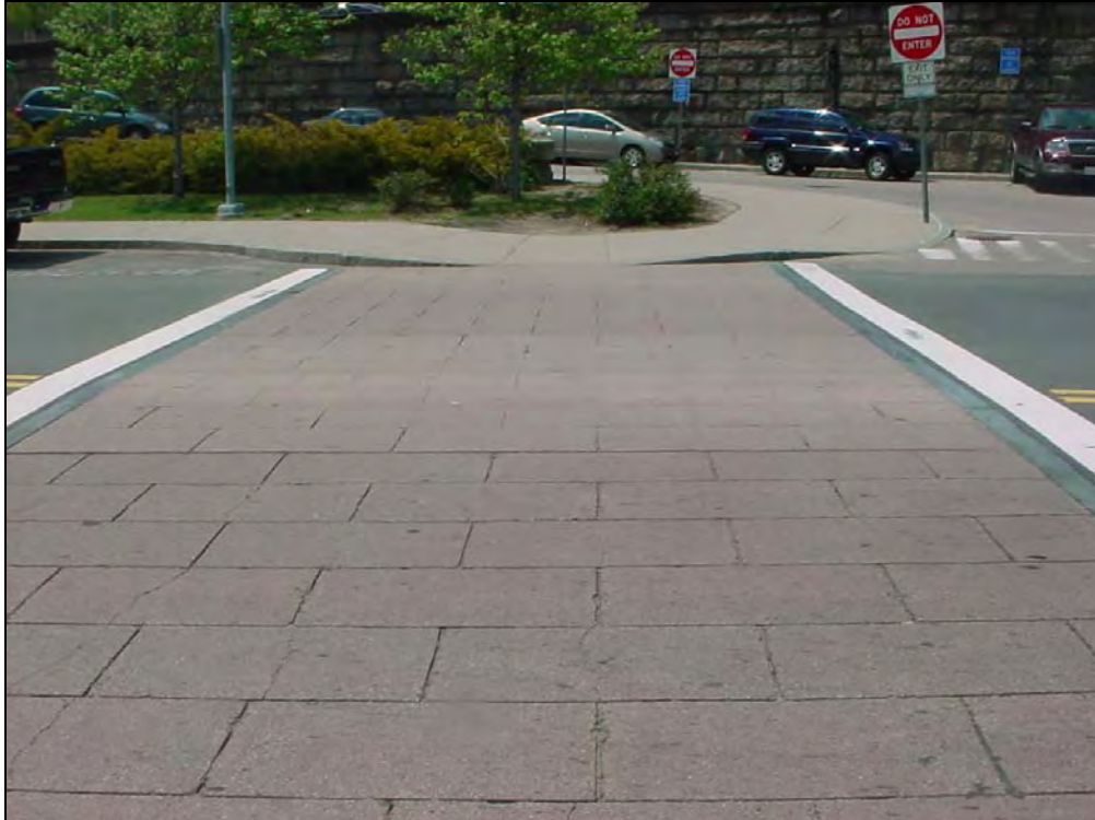
Textured crosswalks Commercial Street, Brockton at Police Station and BAT Centre
