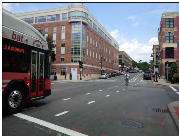
The northbound approach to the Main Street/ Legion Parkway/Centre Street intersection showing post-mounted signals and newly striped bicycle lane (bicycle lanes within the intersection should be painted green).
