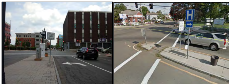
Existing Legion Parkway median on the left lacks pedestrian refuge (the crosswalk is outside the median) and is not wheelchair accessible. The median on the right is an example of wheelchair accessibility at a median from the Main Street/Plain Street/Keith Avenue intersection, Brockton.
