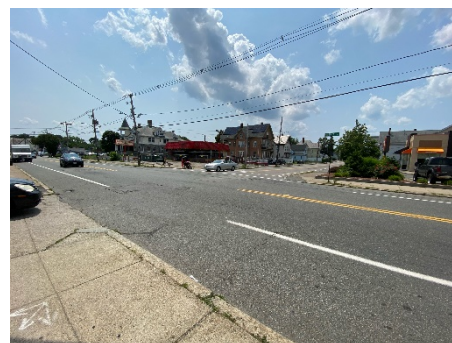
Image 2: There are no drainage or stormwater facilities at the intersection.
