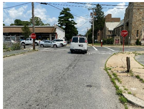
Image 1: Vehicle entering from side streets (view from Nilsson Street eastbound approach).
