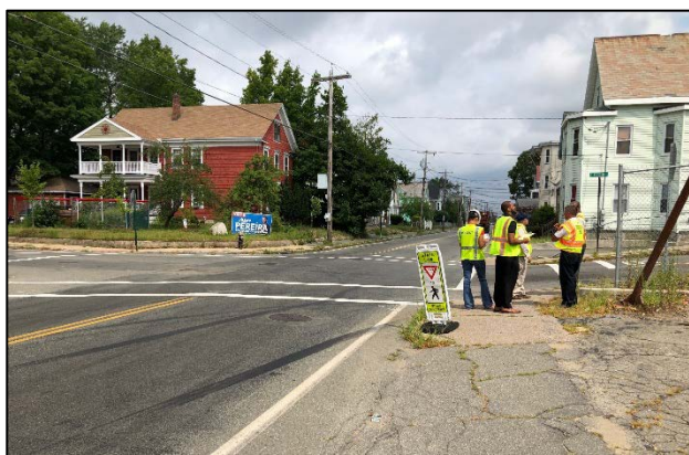
Vegetation on the northwest corner of the intersection (next to a house on the corner) blocks sight lines for East Nilsson eastbound vehicles.
