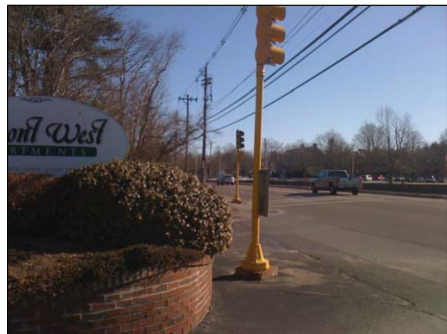
Unprotected signal post and limited sight lines at Belmont Court.
