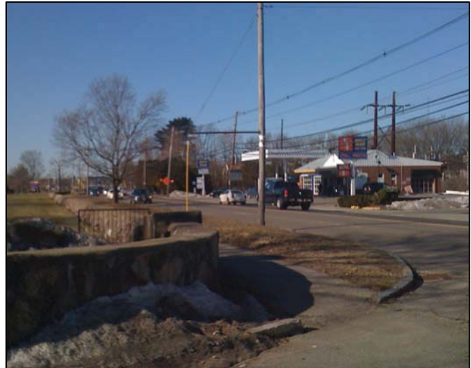
Stone wall along south side of Belmont Street.
