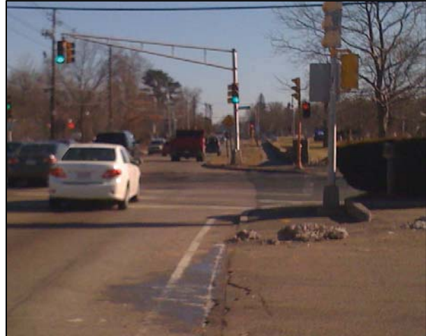
Offset alignment along Belmont Street eastbound.
