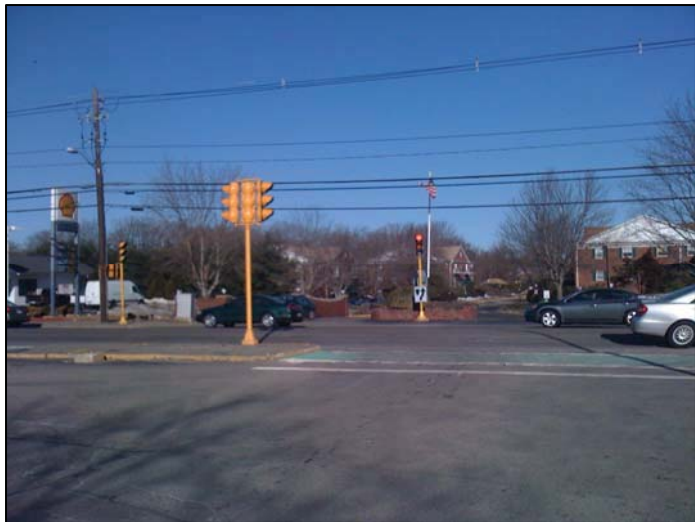
Median islands on side streets result in wide intersection along Belmont Street.
