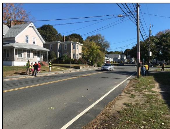
Vehicle taking a left turn from Thatcher Street to Pine Street crossing the double yellow line encroaching on the Pine Street eastbound approach lane.
