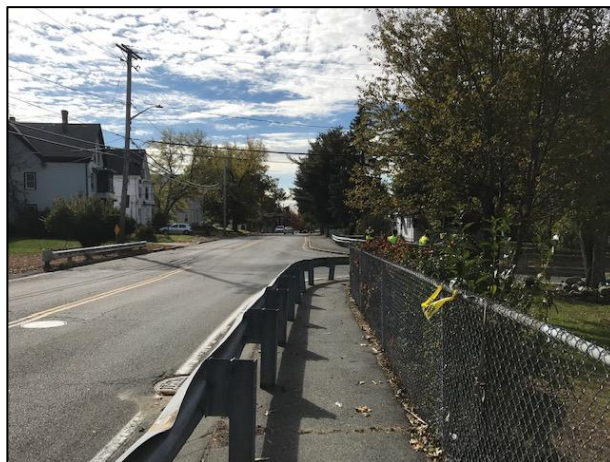
The North Cary Street southbound approach to the North Cary Street/Ames Street intersection.
