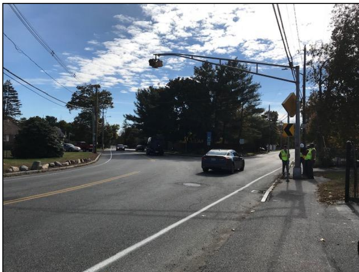
The southbound North Quincy approach to the North Cary/North Quincy intersection, showing overhead flashing beacon, chevrons, and flashing warning signs (facing vehicles approaching from North Quincy westbound).
